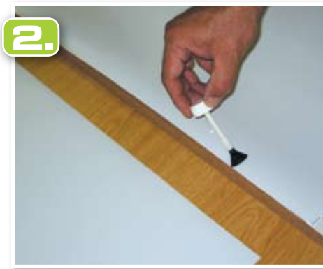
1. Simply spread the PVC weld along the area supported by the Meranti.
