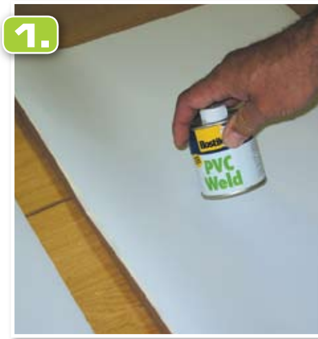
1. Simply spread the PVC weld along the area supported by the Meranti.
